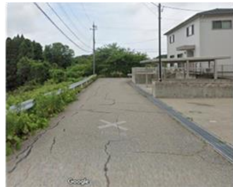
(a)盛土崩壊前
