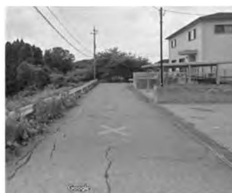
(a)盛土崩壊前
